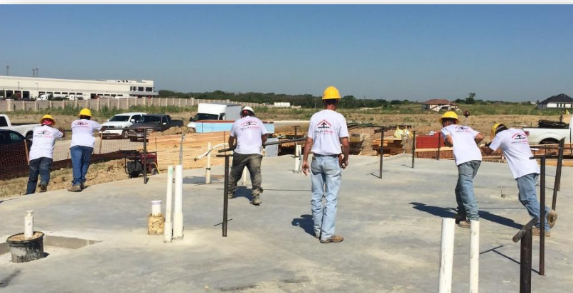
SlabTek Crews Lifting the Foundation
