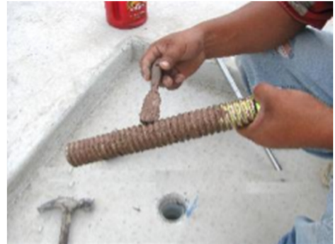
Lubricating lifting bolt threads
