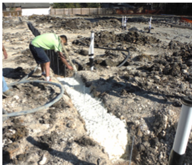
Suspended Plumbing with light-weight material covering plumbing prior to the slab pour and slab lift
