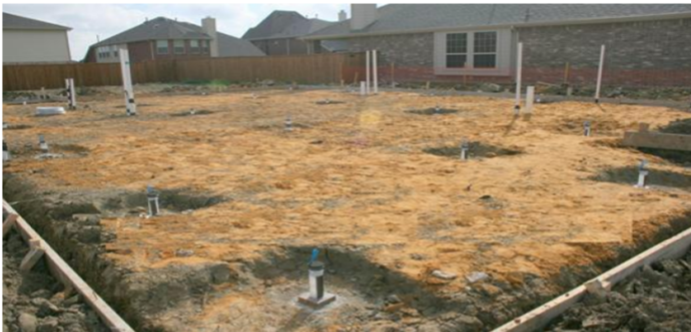
Piers, Mechanisms, Capitals, Perimeter Beams, Pad prepared – ready for installation of reinforcement
