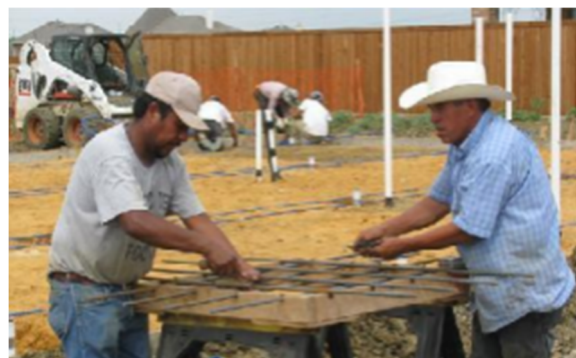
Rebar grid being formed using jig
