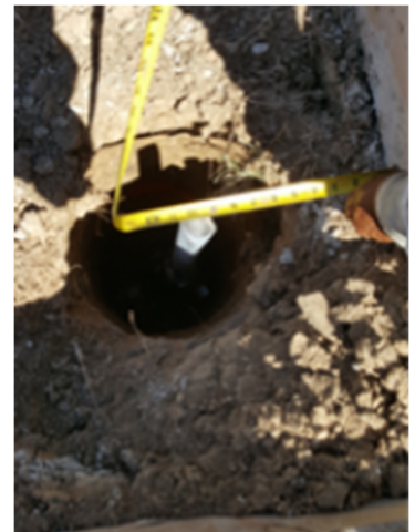
The helical pier is measured to assure it is center and cut to the proper height
