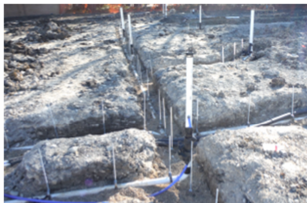
Suspended Plumbing with Threaded Rod
