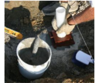
Mech installed using epoxy
