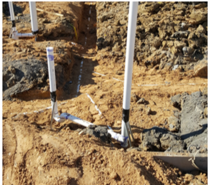
Plumbing Installation using Cushion Sand
