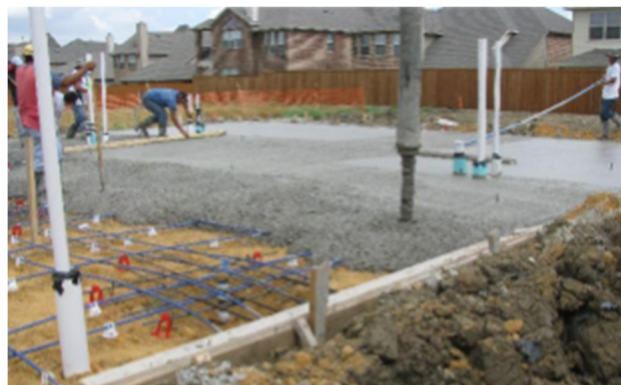
Placing concrete on the prepared pad
