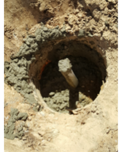
Concrete Cap Poured around Helical Pier top
