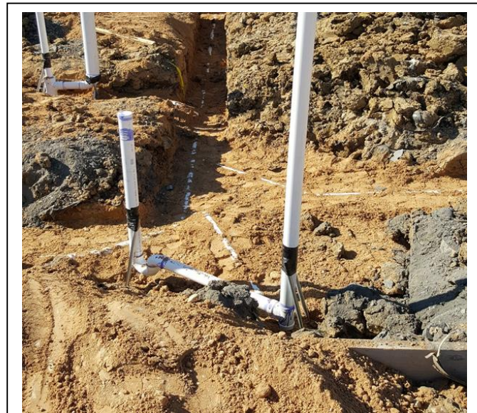
Plumbing Installation using Cushion Sand
