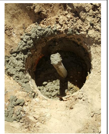
Concrete Cap Poured around Helical Pier top
