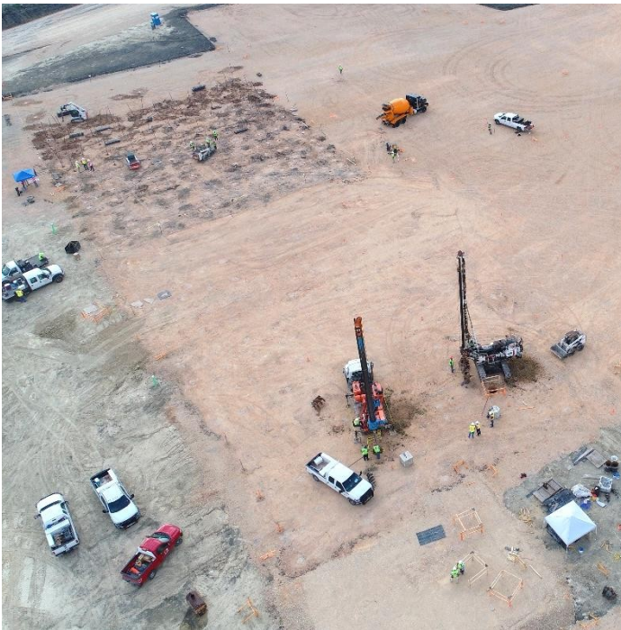
Helical Piers installed together with heavy concrete piers used to carry the structural load while Helical Piers carry the slab load.
