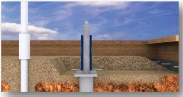
1. The Lifting Mechanism is set on the pier during slab make up. The slab is thickened at the pier for added strength.
