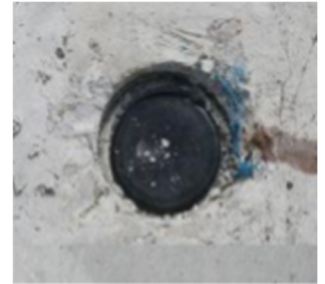
Finish cap installed
