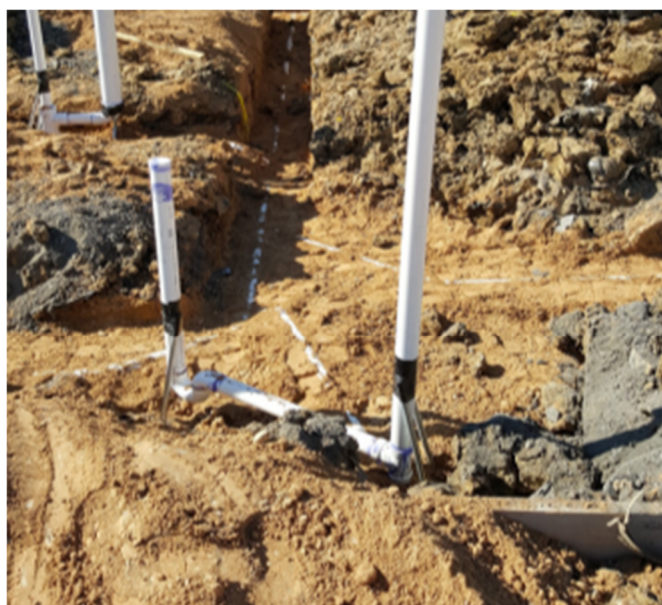
Plumbing Installation using Cushion Sand
