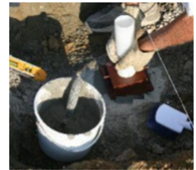
Mech installed using epoxy
