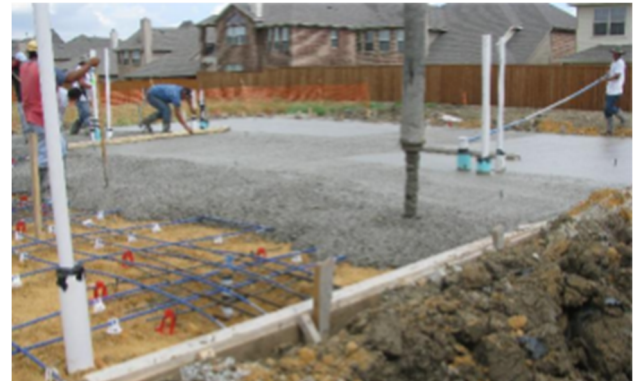
Placing concrete on the prepared pad
