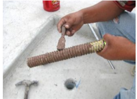
Lubricating lifting bolt threads
