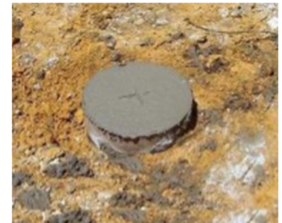
Pier top ready for Mech
