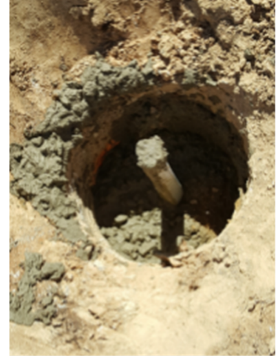
Concrete Cap Poured around Helical Pier top
