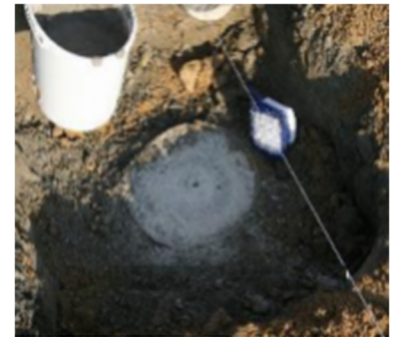
Hole for dry Mech Install
