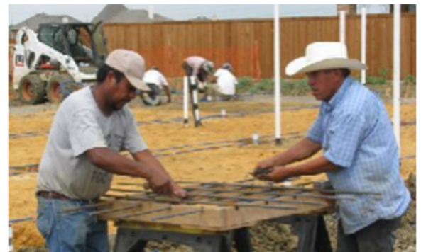
Rebar grid being formed using jig
