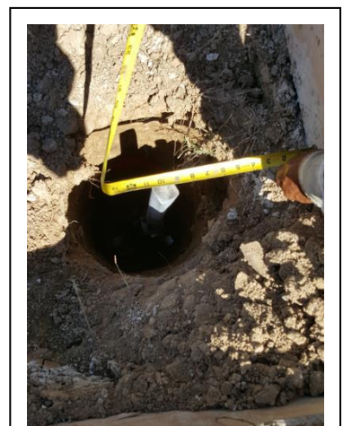
The Helical Pier is measured to assure it is center and cut to the proper height
