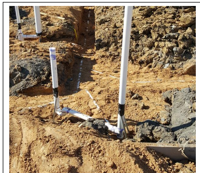
Plumbing Installation using Cushion Sand
