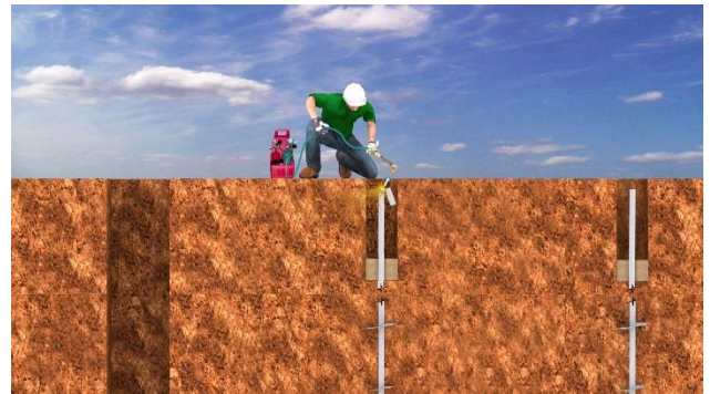
2. Helical Pier Cut to Proper Height
