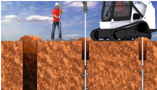
1. Helical Piers Installed
