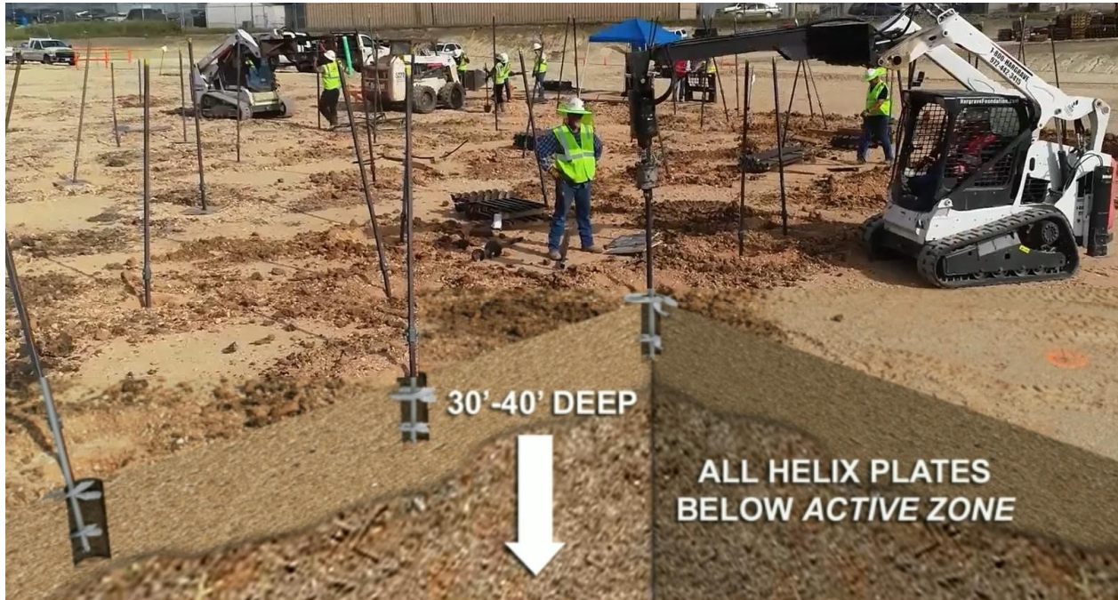
SlabTek installation crew carefully monitors the Helical Pier Angle, Depth, and Torque
