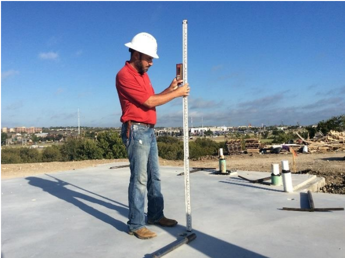
Elevations are Taken at Each Pier Location
