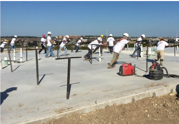
Slab is raised 1/3" per Bolt Rotation
