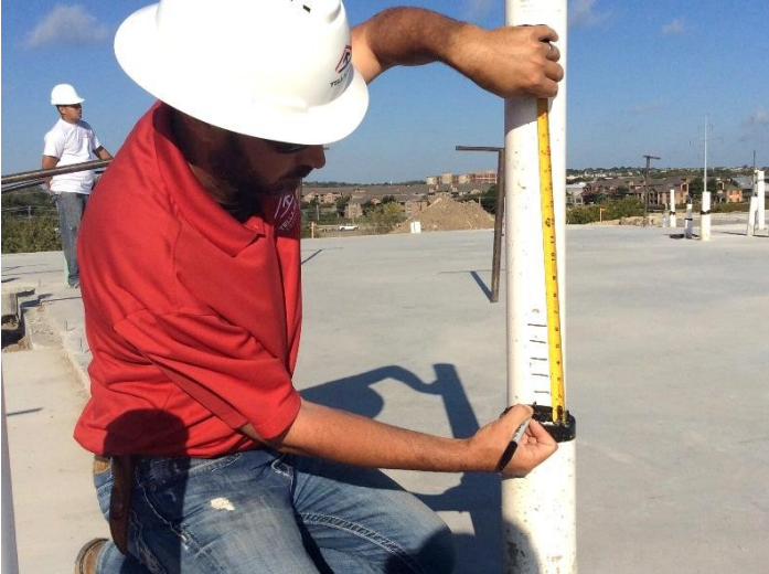
Plumbing is Marked and Carefully Monitored
