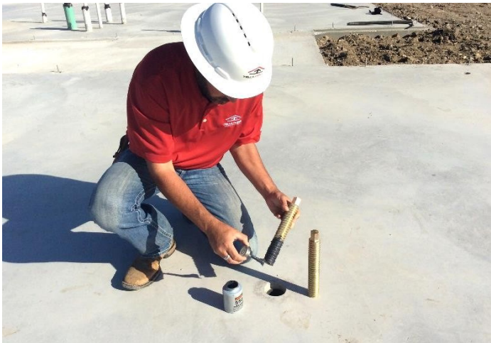
Lifting Bolt Greased and Installed
