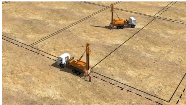
Drill truck drilling 18" and 24" diameter piers
