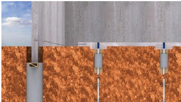
Wall panels in place, ready for the slab to be lifted
