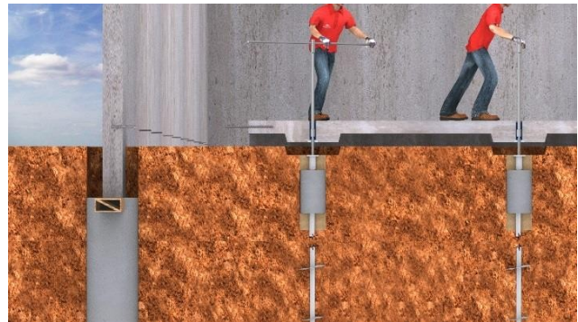
Slab lifted to create protective void under the slab
