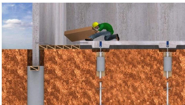
Carton forms are placed in the pour strip area
